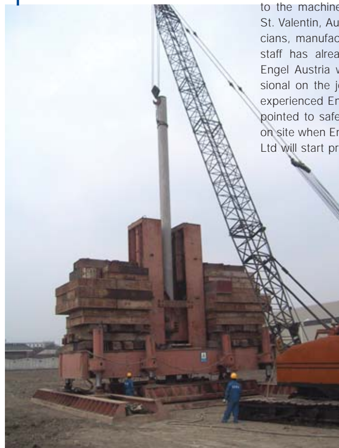
With the force of 800 ton piles were driven into the ground.
